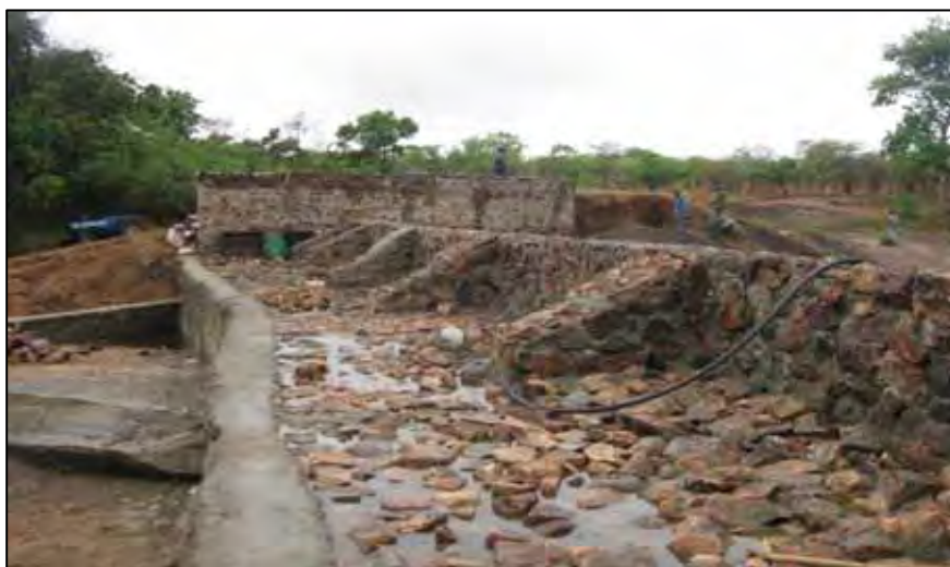
Construction of a dam to provide a permanent water source for wildlife in Coutada 9
